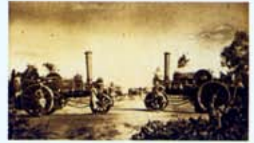
Road Rollers ready to go into operation — Sakchi, 1909.
